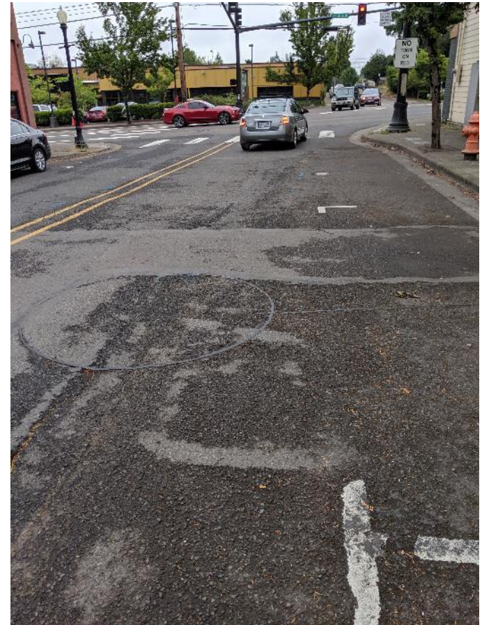
Loop in close proximity to parking spot (WB approach)
