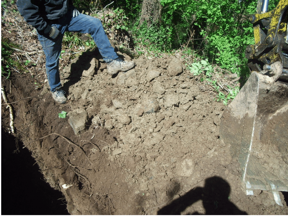
Photo 5 - Spoils from test pit TP-3.
