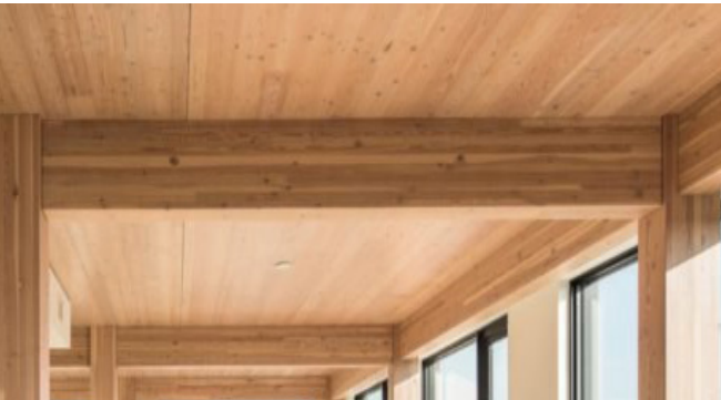
CROSS LAMINATED TIMBER (CLT STRUCTURE INTERIOR VISIBLE FROM EXTERIOR THRU GLAZING)
