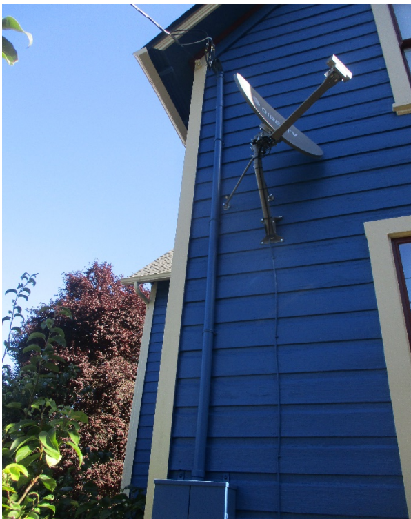
Meter Conduit (for visual of where our conduit will run)
