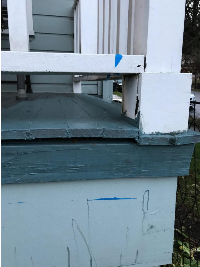
Figure 3. Porch materials to be replaced. The wood has been recently painted in an effort to protect it from the weather until it is replaced.
