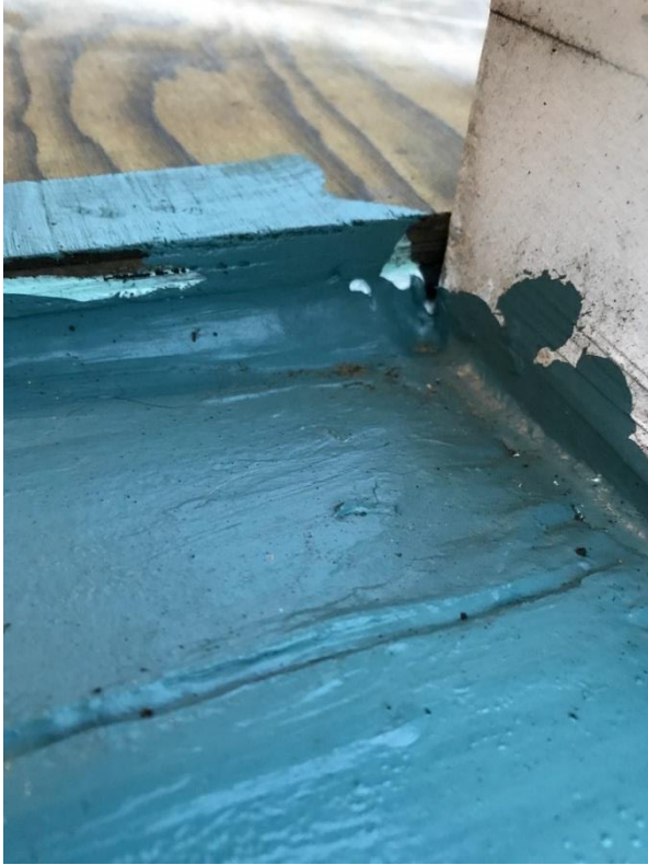
Figure 5. Porch materials to be replaced. Plywood is covering a hole in the porch floor. The wood has been recently painted in an effort to protect it from the weather until it is replaced.
