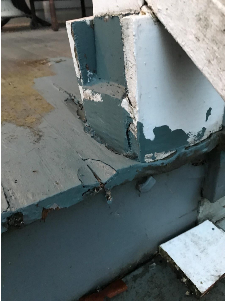
Figure 4. Porch materials to be replaced. The wood has been recently painted in an effort to protect it from the weather until it is replaced.
