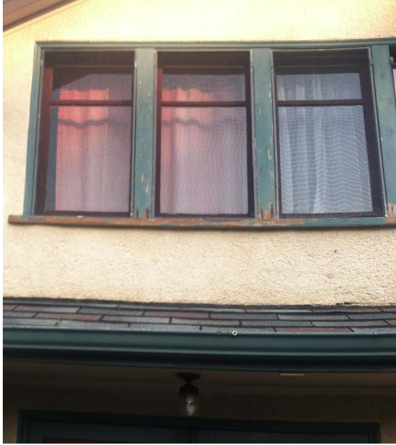
Framing around house windows to be refurbished
