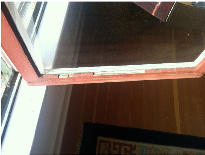
Caulking around window to be refinished
