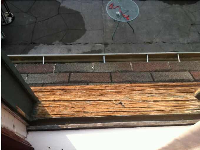
Framing around window to be refinished
