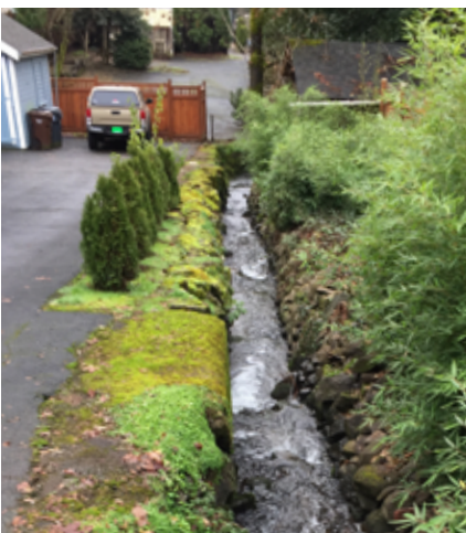
Retaining walls along chanelized man made stream for rainwater runoff
