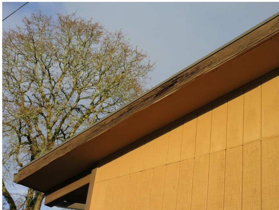
Figure 6: Fascia Damage
