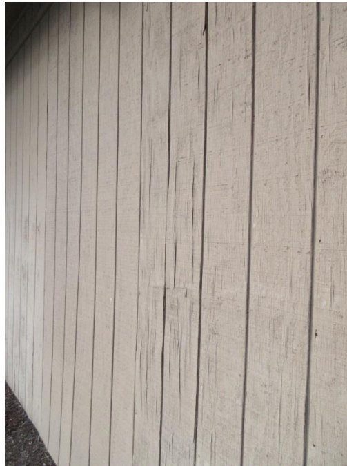
Figure 3: Siding Damage
