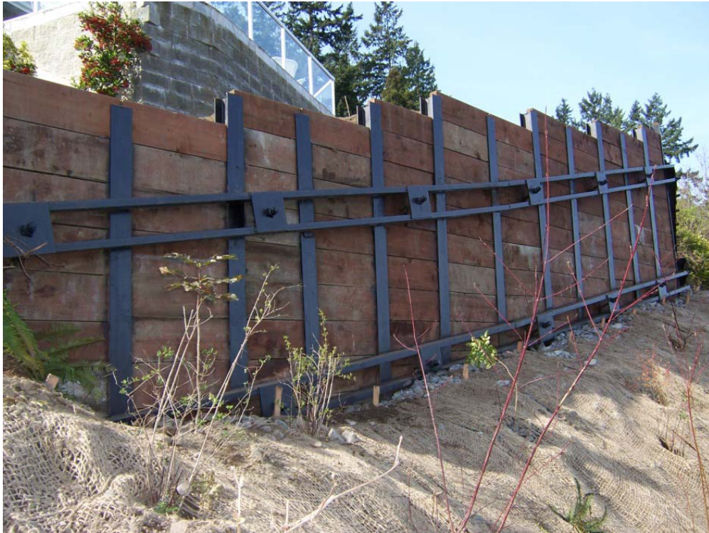
Sample Soldier Pile and Tieback Wall with Wood Lagging and Waler System
