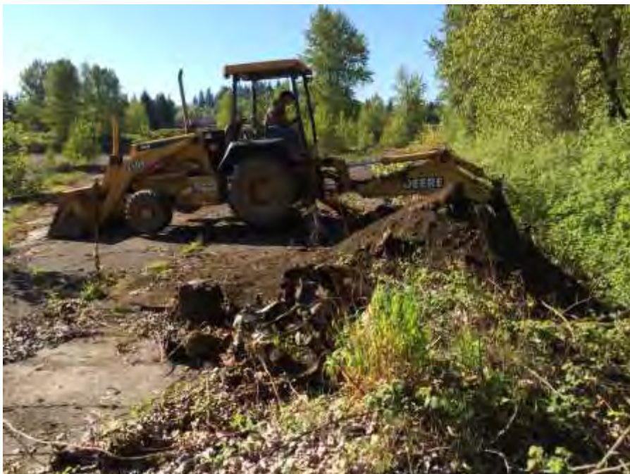
Facing South, Test Pit TP-3, Excavating Fill and Garbage
