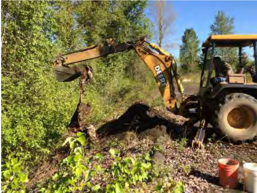
Facing North, Test Pit TP-3, Excavating Fill and Garbage
