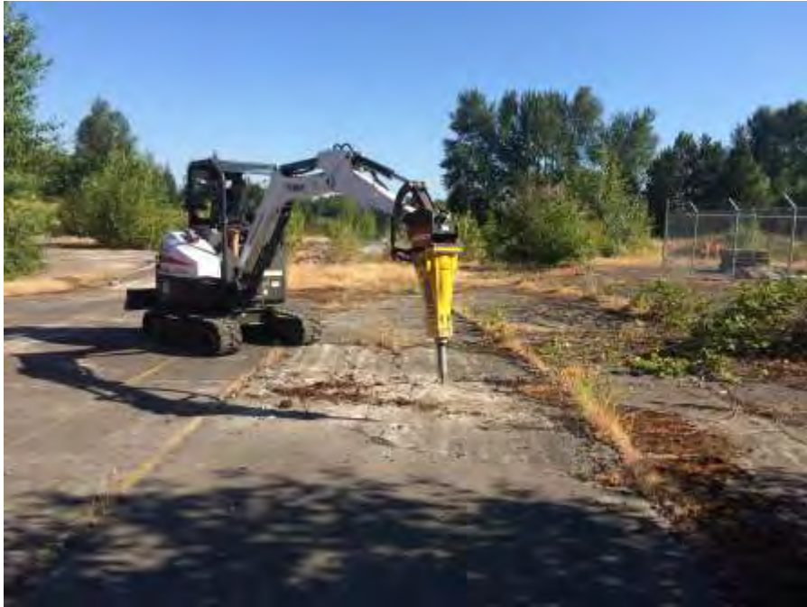
Hydraulic Rock Chipper Used to Penetrate Concrete Fill
