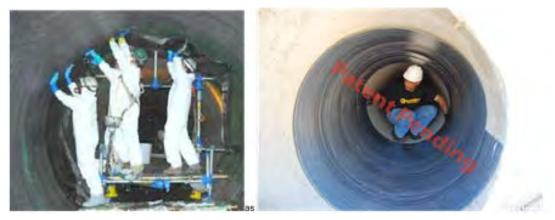
Figure G-5. Examples of pipe wrap installation
