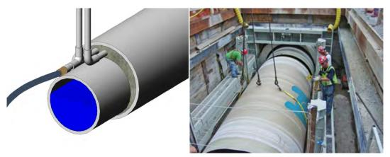
Figure G-4. Examples of sliplining installation
