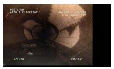
Figure G-11. Video image from laser profile inspection
