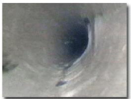
Figure G-6. Examples of cured-in-place point repair
