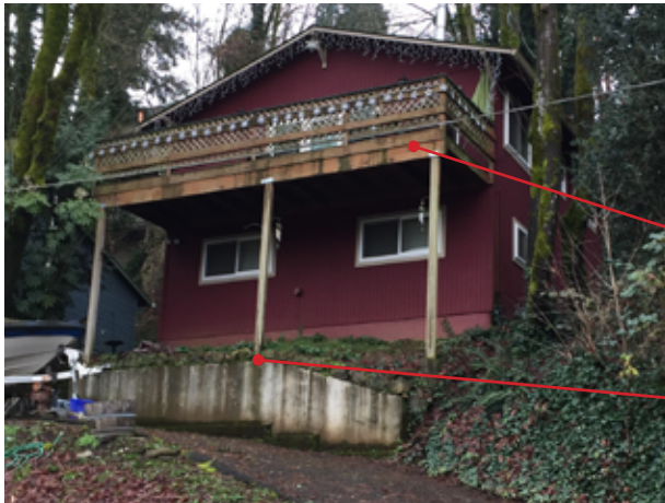
Upper level balcony covering first level
