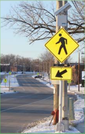
Multiple Solar-Powered beacons flash in unison, wirelessly synchronized by BlinkSync technology
