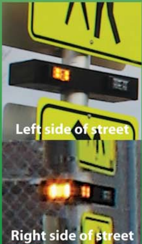
Multiple Solar-Powered beacons flash in unison, wirelessly synchronized by BlinkSync technology
