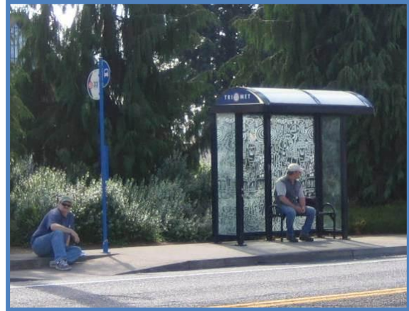
Additional transit stops with shelters would encourage more people to take transit.
