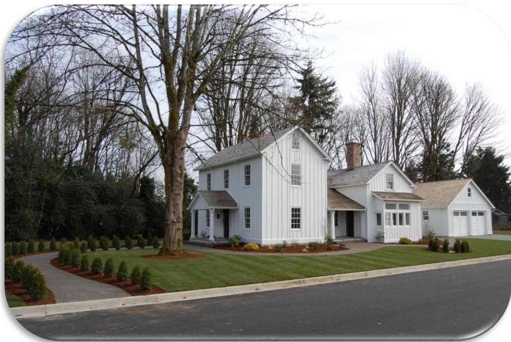
McCarver House 2008- New garage and kitchen addition
