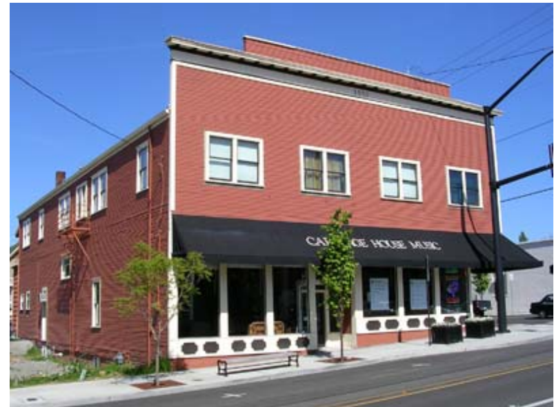
2 Story Historic False Front
