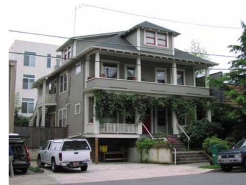
2 ½ Story Four Square Multifamily
