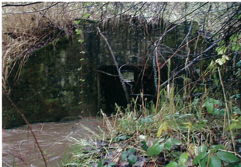
From culvert inlet opening, looking downstream through the 6'x 6' concrete box culvert
