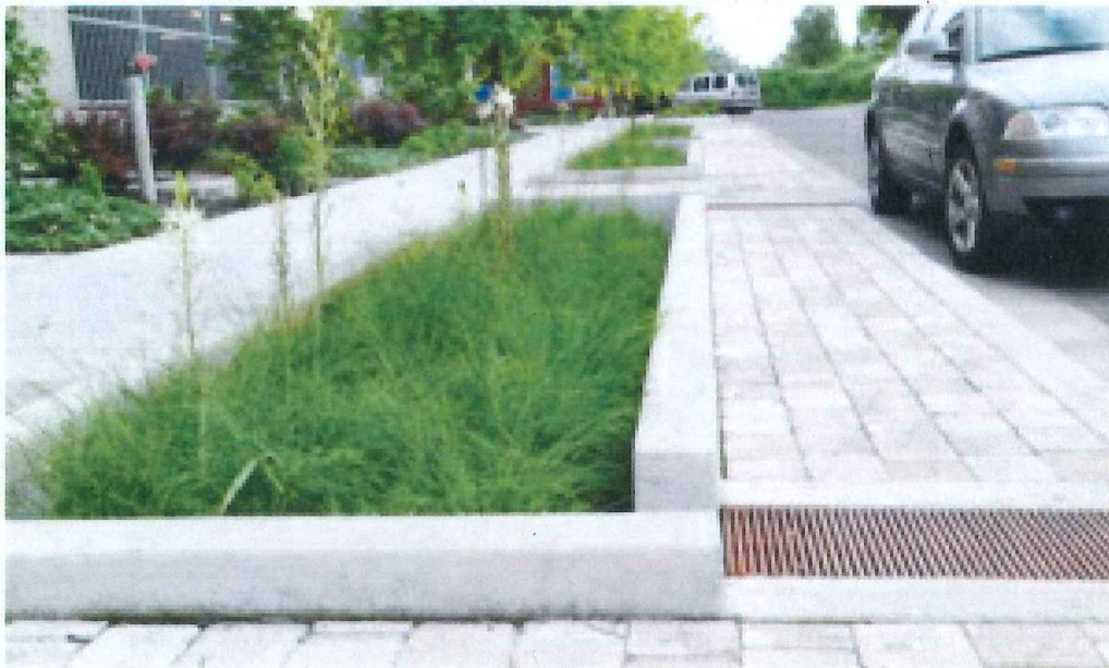
Beaumont Village Lofts, NE Portland
