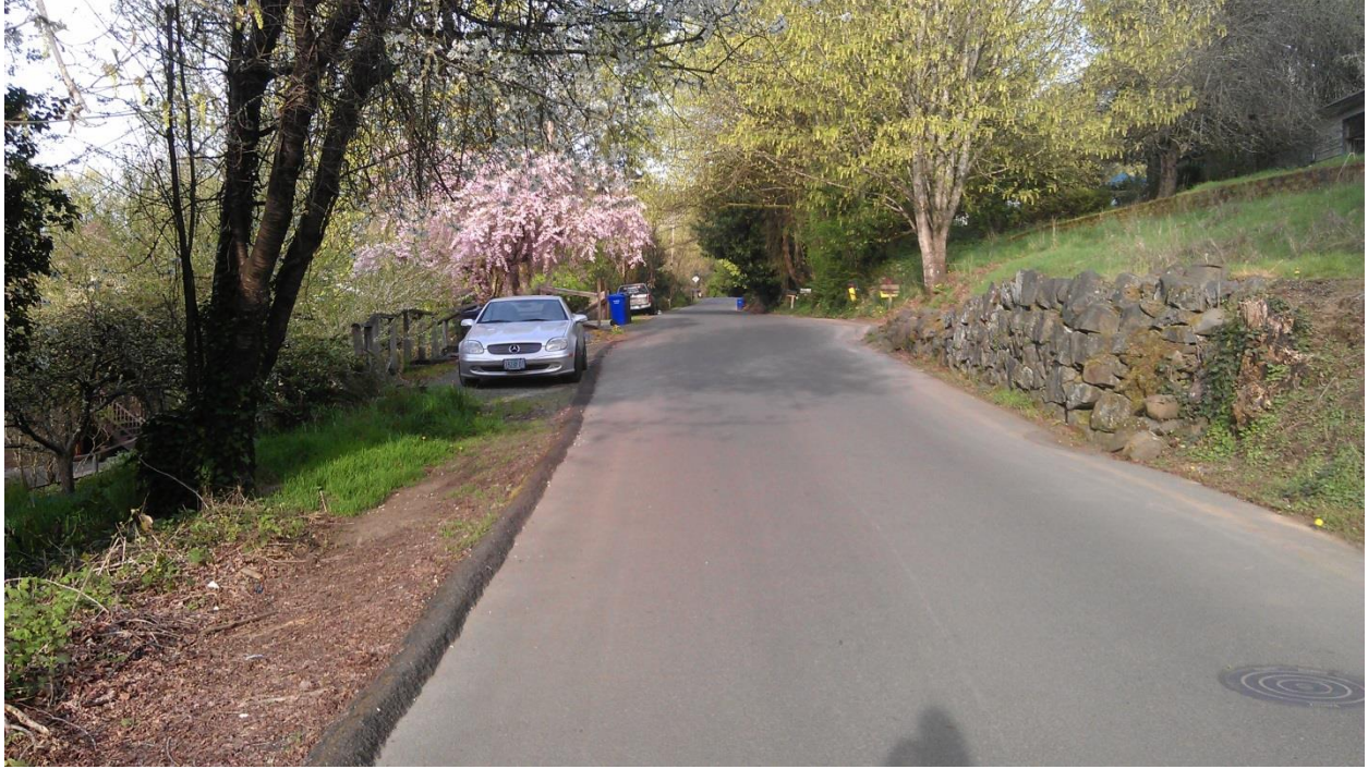
At 4 th Street looking East
