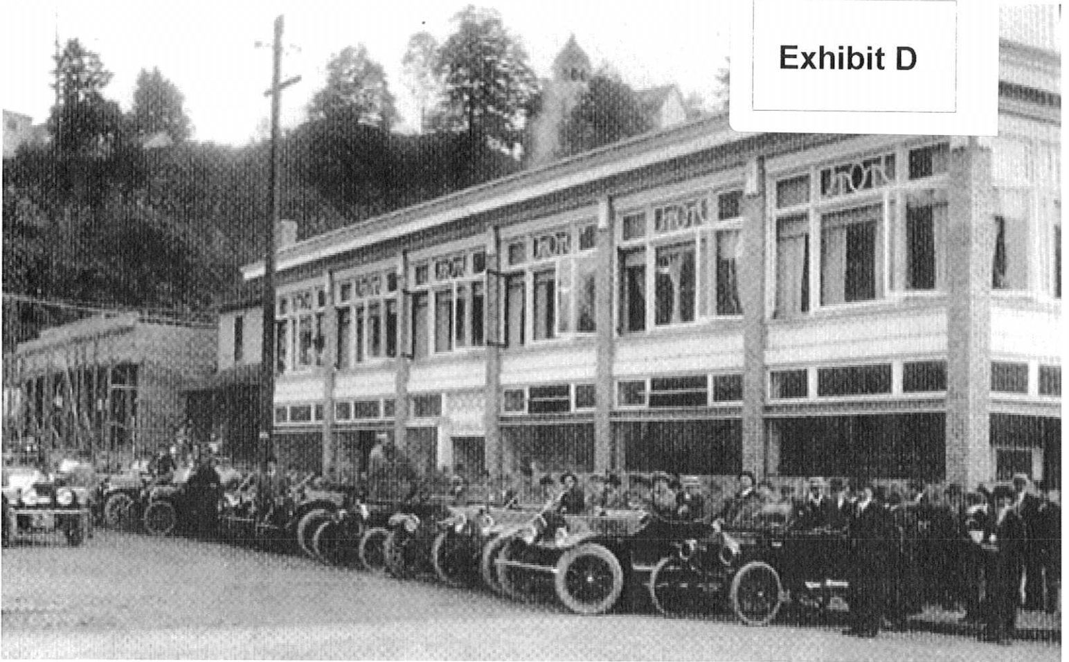
722 MAIN STREET STOREFRONT IMPROVEMENT PROGRAM April 26, 2013
