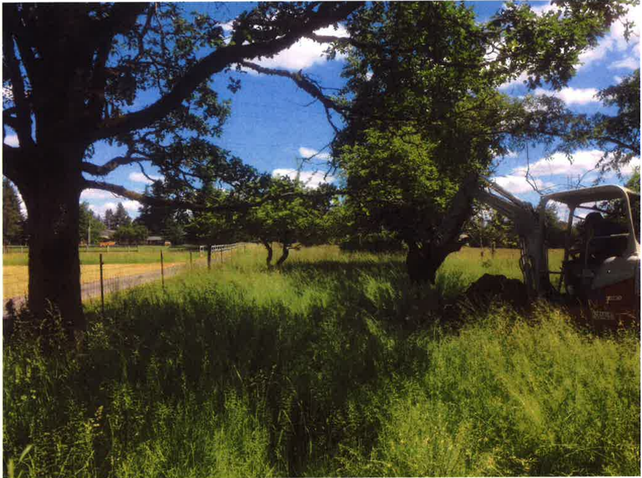
Test Pit TP-5, view to the North
