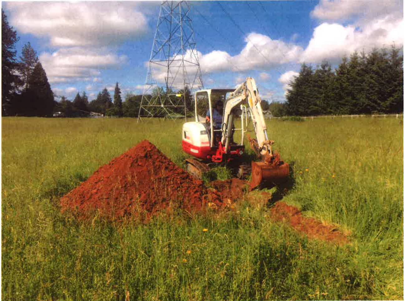
TP-3, 19701 Leland Road, view to the southwest
