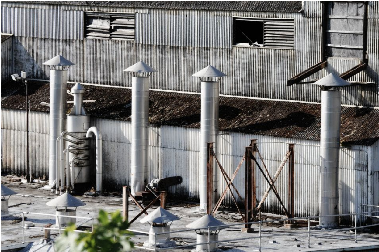
Chimneys at Mill C.
