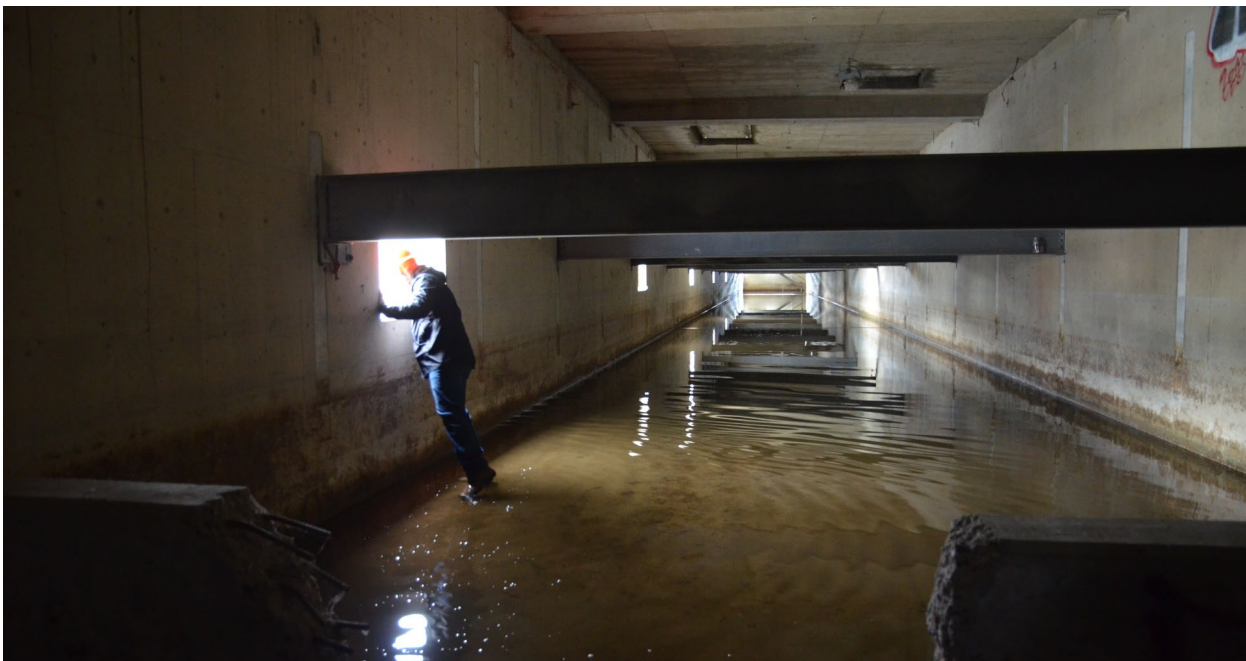
Inside the Pipe Chase
