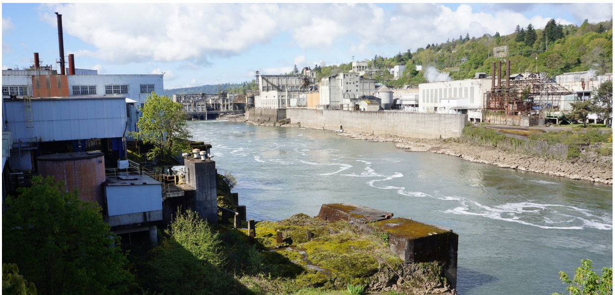
Upper Right: Oregon City Municipal elevator
