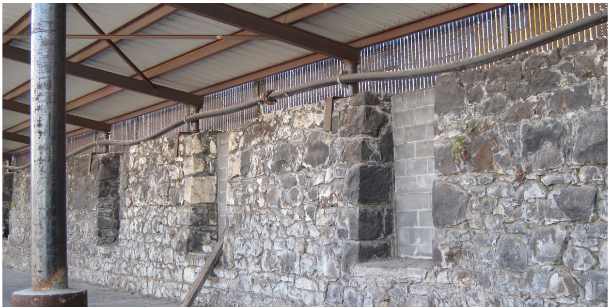
Woolen Mill basalt stone foundation walls
