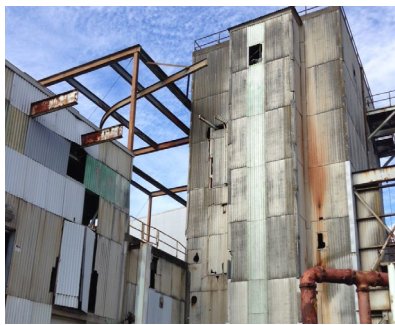
Mill H building
