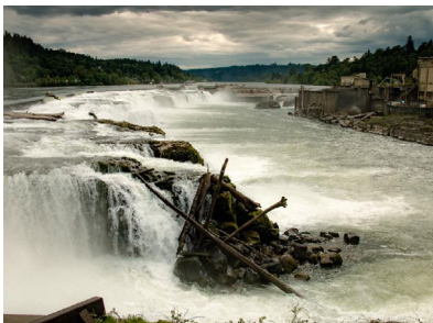
View from the Hawley Powerhouse Foundation
