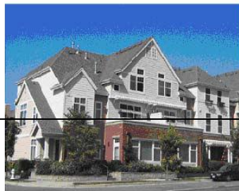
This multifamily building uses a combination of horizontal and vertical modulation, roofline modulation, distinctive window patterns, and clear articulation of the building's top, middle, and bottom to help reduce its perceived architectural scale and add visual interest.
